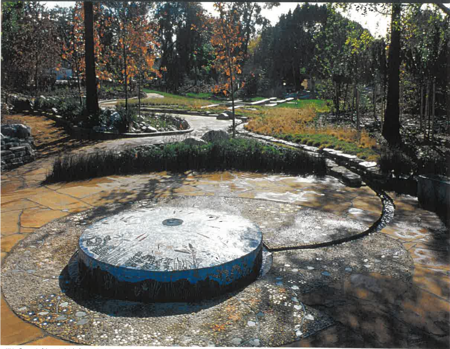
Water flows out of the central eight-foot circular disk in the plaza at the uppermost corner of the site. The plaza is paved with random flagstone and furnished with two, poured-in-place concrete seat walls. Planting includes indigenous trees, ornamental grasses, lavender, and California poppies.
